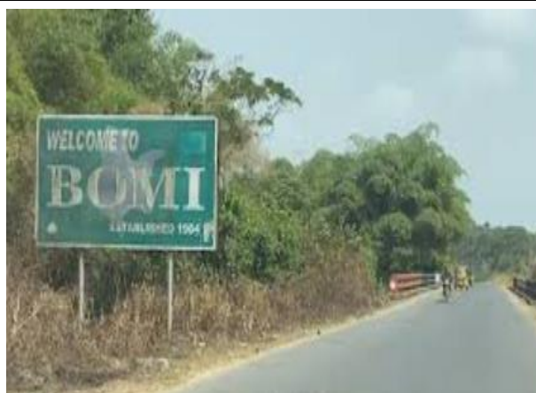
Figure 17: View of the road condition at Po River bridge
