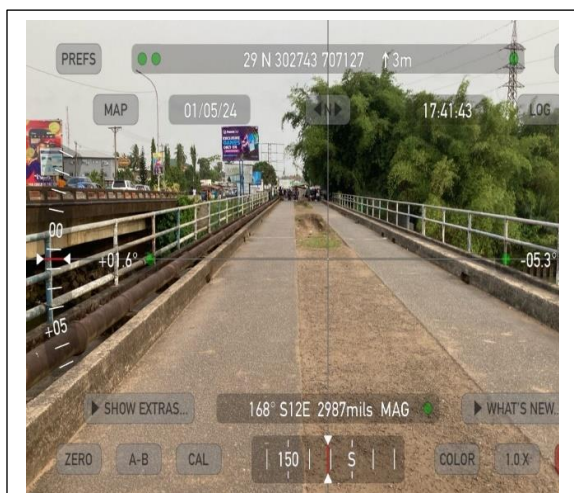
Figure 15: St. Paul Bridge Rail side (b)
