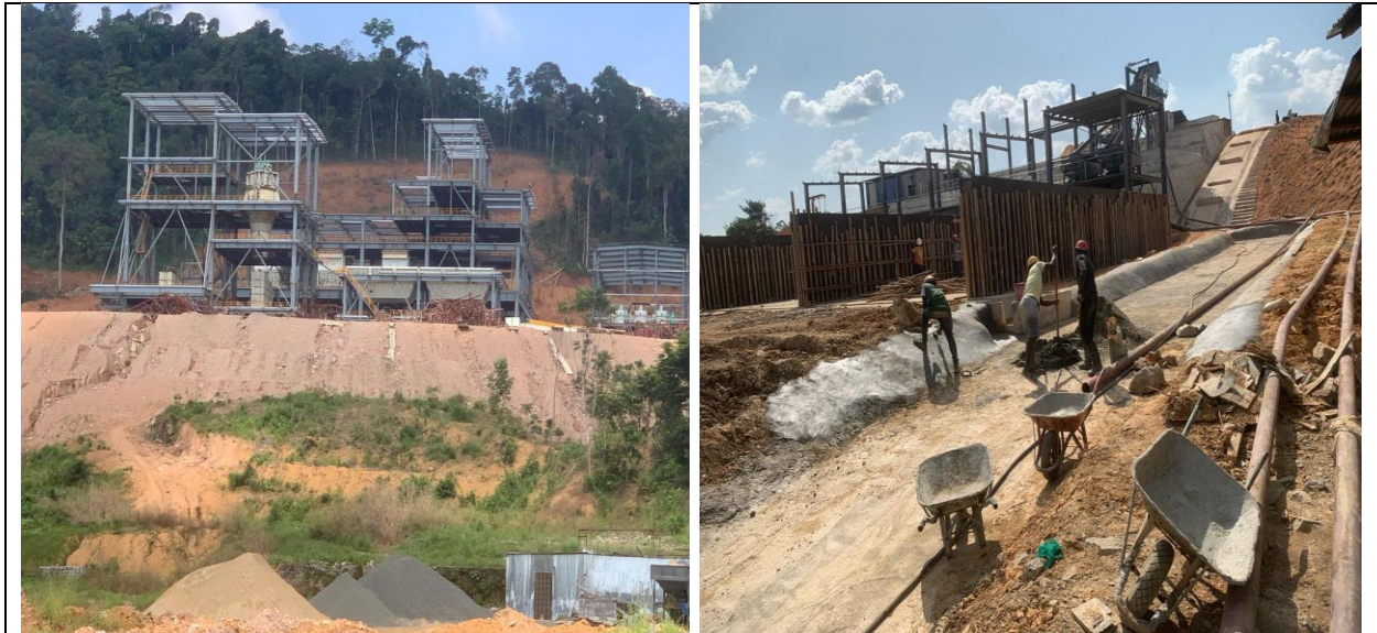
Construction of new Beneficiation Plant at the Mines left and New TSF
